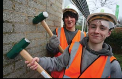
Countesthorpe Community College students Will Attfield (front) and Lewis Sreaton (rear) preparing to demolish the bungalow.
